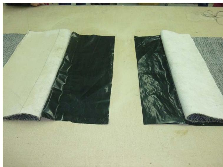
2. The Geomembrane of the left panel shall be covered with Geomembrane of the right panel, creating overlap.
