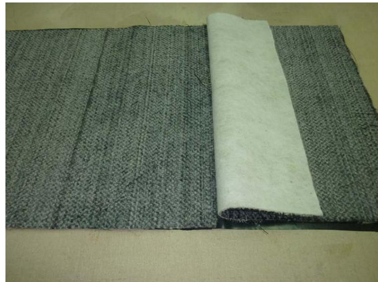
4. The bentonite shall be poured on the edge of one panel (in this case left one).
